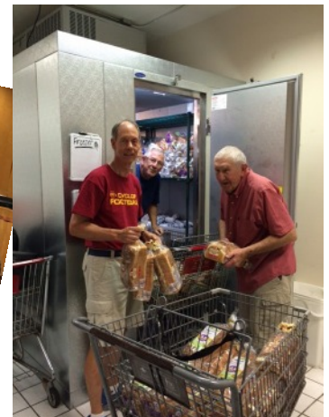
Walk-in Freezer, Burk Foundation Grant
